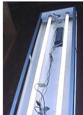
Electrical hazards may also be found in light fixtures. Uncovered fluorescent lights, incandescent light fixtures without bulbs, or light fixtures hanging by wiring are all dangerous. Fluorescent lights have energized wiring, starters, and ballasts under their protective covers. If the light's cover is not properly replaced, these hazards are exposed.
