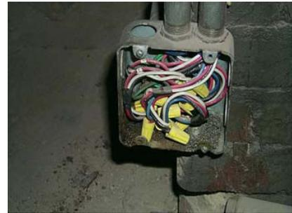
When energized junction boxes are uncovered, the wiring is vulnerable to damage and accidental contact. If easily combustible materials, such as paper or cardboard, are stored near unprotected energized wiring, a spark or electrical arc could easily start a fire.
