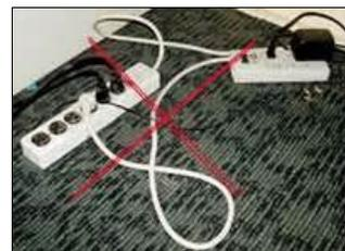
sion cords are to be used temporarily and never as a permanent source of power to equipment.
